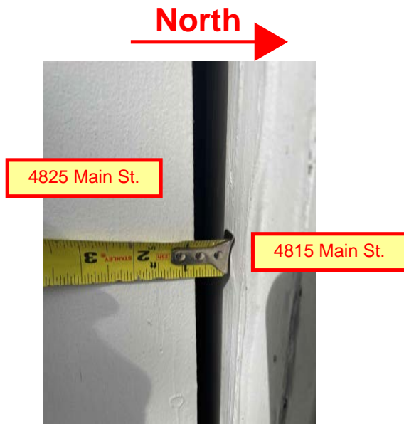
Structural Separation at South Face Exterior Wall (Measured at Front of Building)
