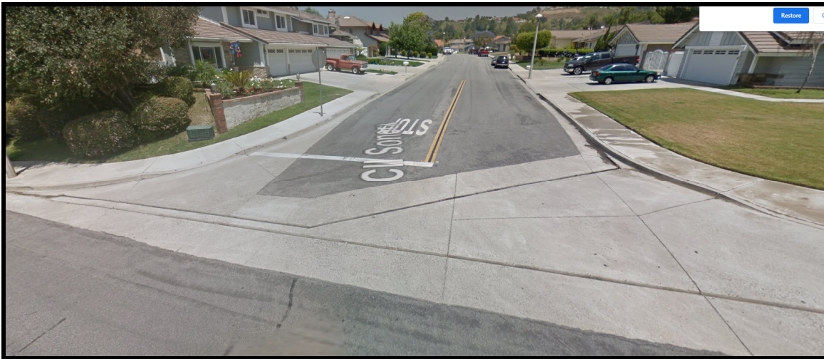
Figure 4: Zone 5 Avenida Adobe and Calle Sonora, PCI 67 – Possible Treatment- Overlay
